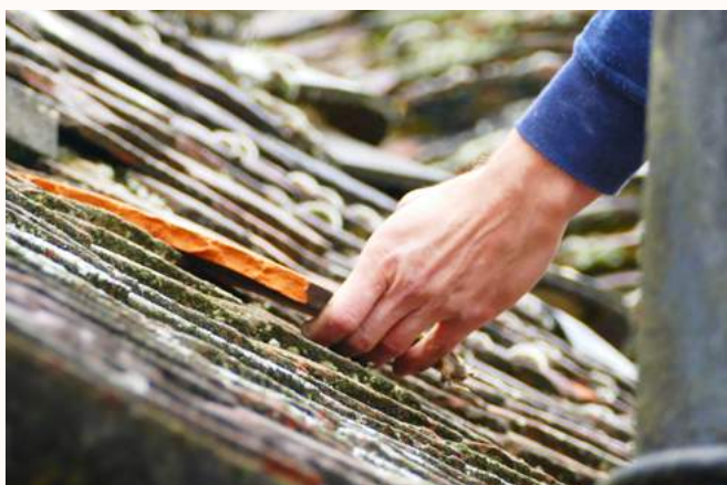
Jane's Fund works to the roof of Jane Austen's House
